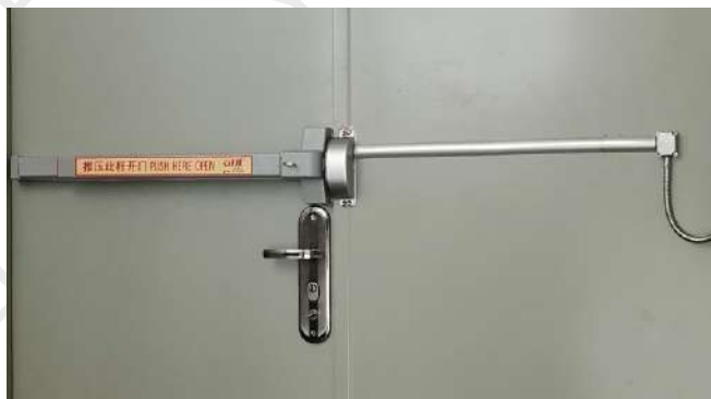
Application scenarios of electric strike with double door push bar device YS-622-S Application diagram
